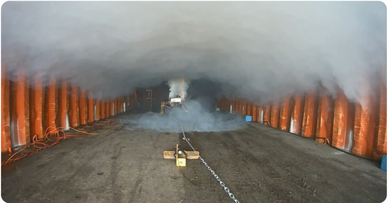
An example of a thermal runaway event with a 1.4kWh lithium-ion battery, 40% state of charge. Large amounts of toxic, flammable vapour fill the confined space. Ref: Christensen, 2023.
